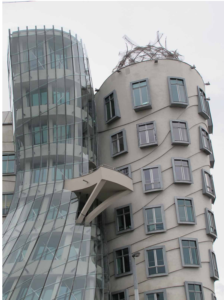
Figure 2. Detail of Gehry's Offices in Praga
