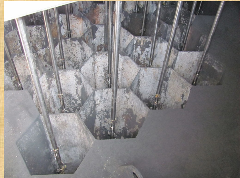
Electrodes inside electrostatic precipitator
